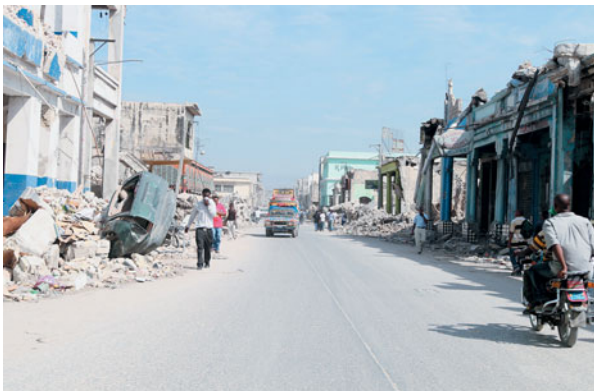
This photograph shows part of the damage in Haiti due to the earthquake of January 2010.
